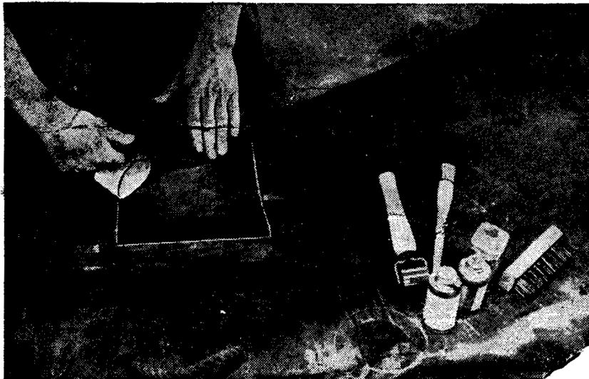
Figure 12. Center the tape over the edge of the patch.
