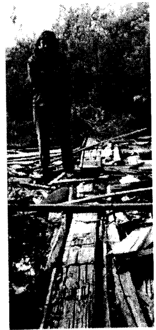
Karla Vander Zanden inspects the blown down house at the homestead.
