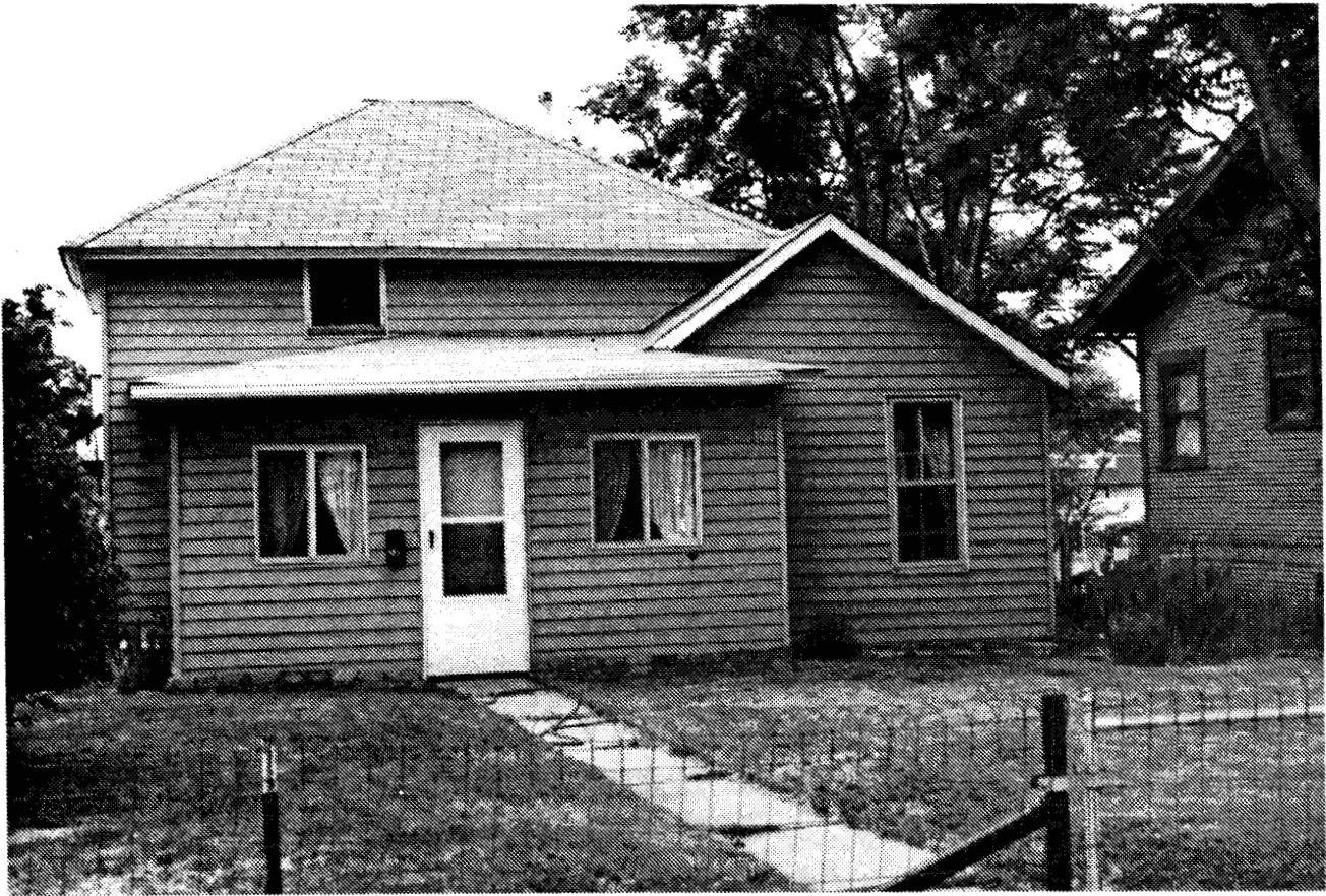
729 Ute Avenue in Grand Junction, CO, as it appears today.
